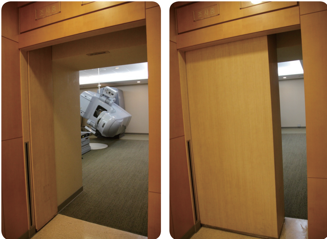
<Opening and closure of the shielding door in the radiotherapy room>
